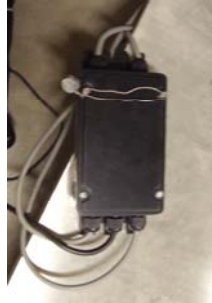
Junction boxes with wire security seals
