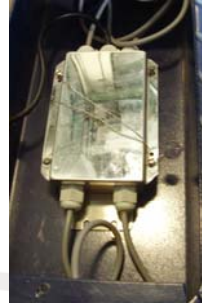
Junction boxes with wire security seals
